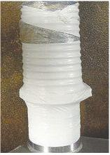
Original connectors were often taped to prevent leakage
