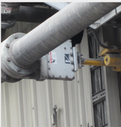
10" (254mm) HDP in-line handling fly ash
